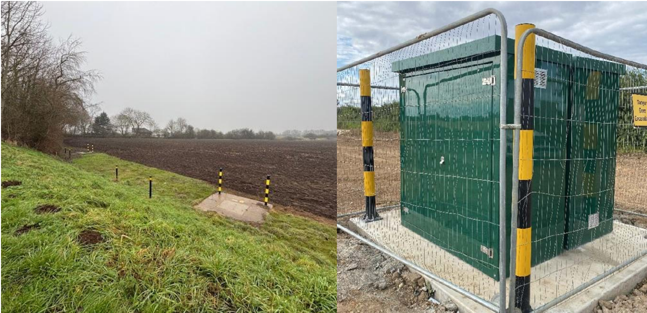
Plate 2-12 Example of an Underground Link Box (Left) ((Source: Dogger Bank A & B) and an Above-Ground Link Box (Right) (Note: This includes temporary fencing during construction) (Source: Dogger Bank B)
