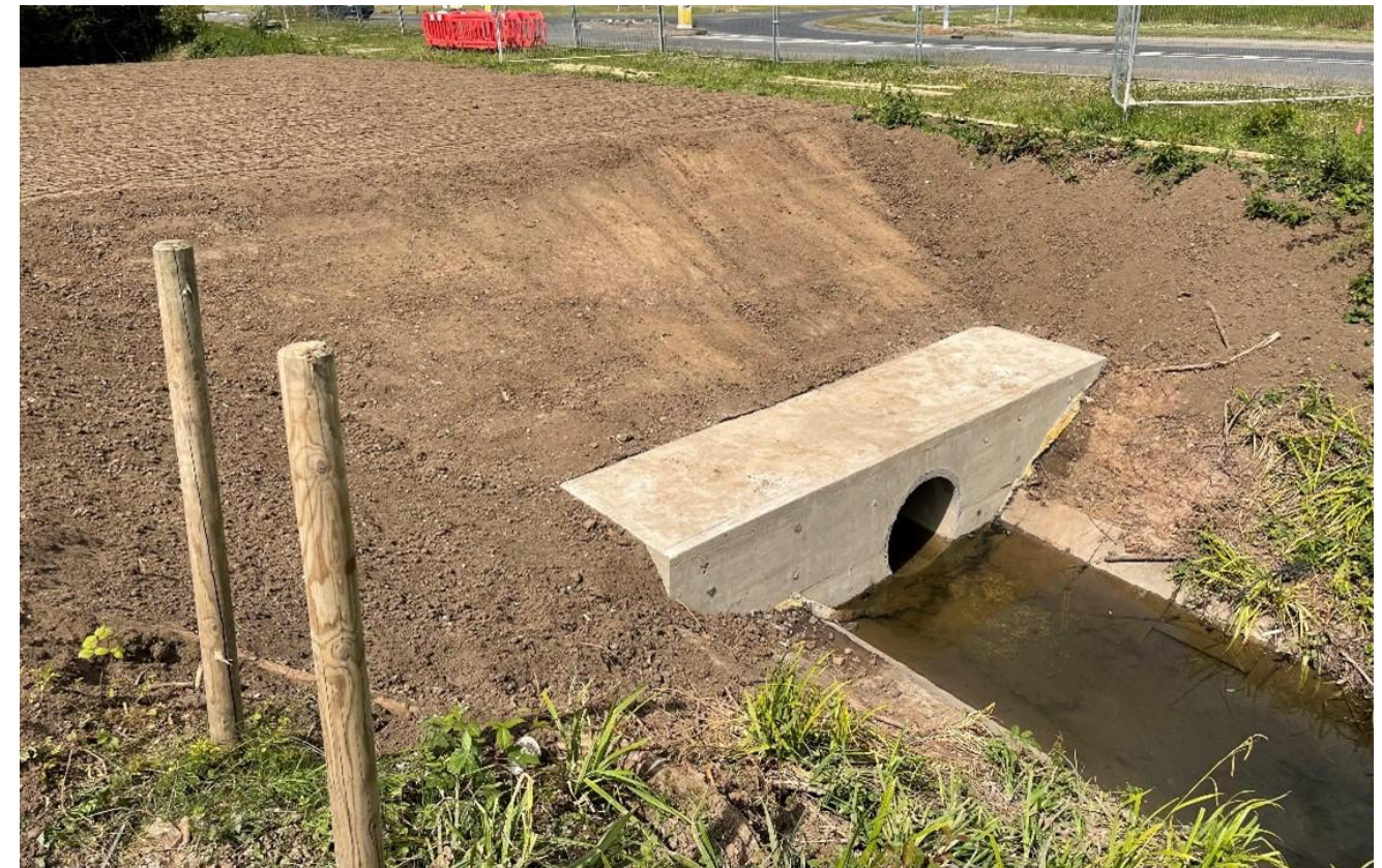
Plate 2-19 Example Temporary Culvert Installation for Minor Water Crossings (Source: Dogger Bank C)
