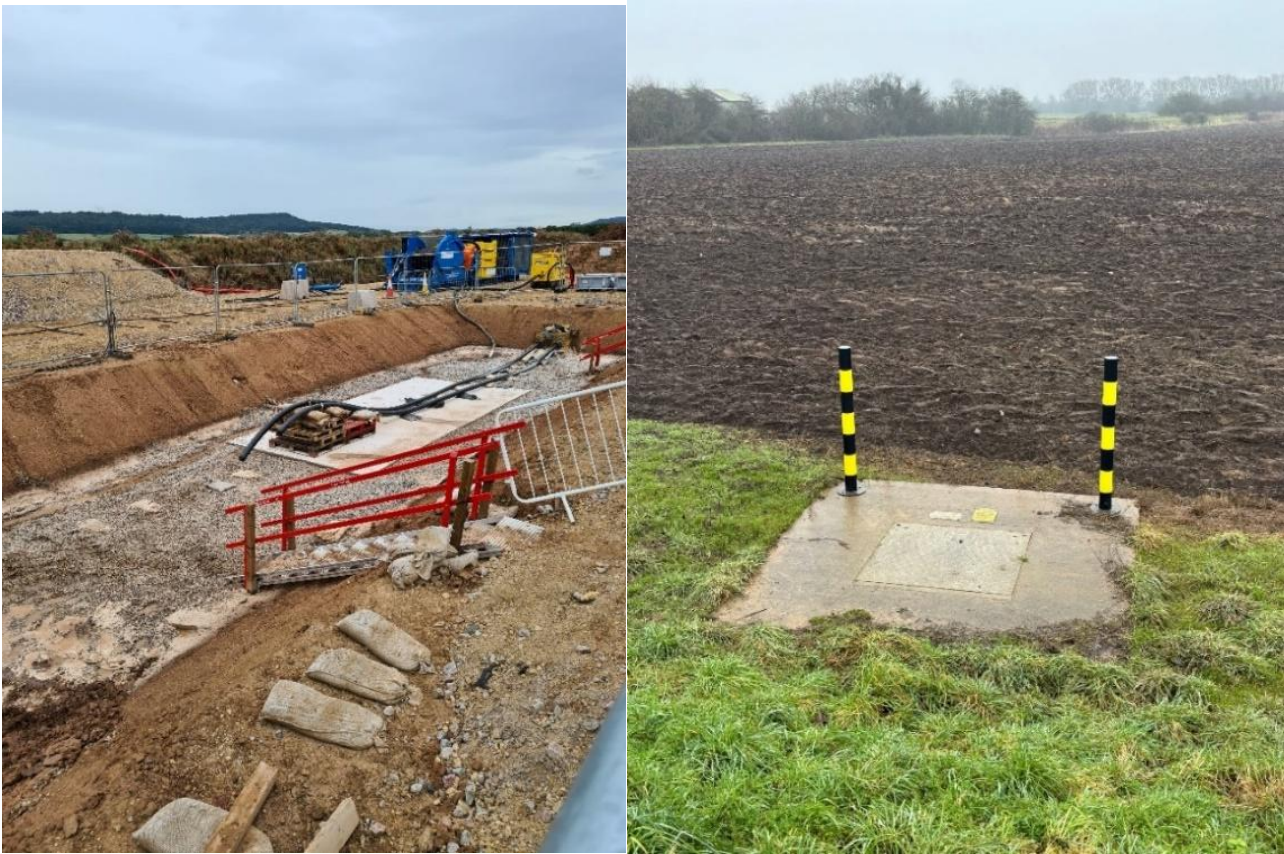
Plate 2-9 Example TJB during Construction (Left) (Source: Dogger Bank C) and Example Underground Link Box during Operation (Right, Note: Only manhole cover to the underground link box will be visible at ground level) (Source: Dogger Bank A & B)
