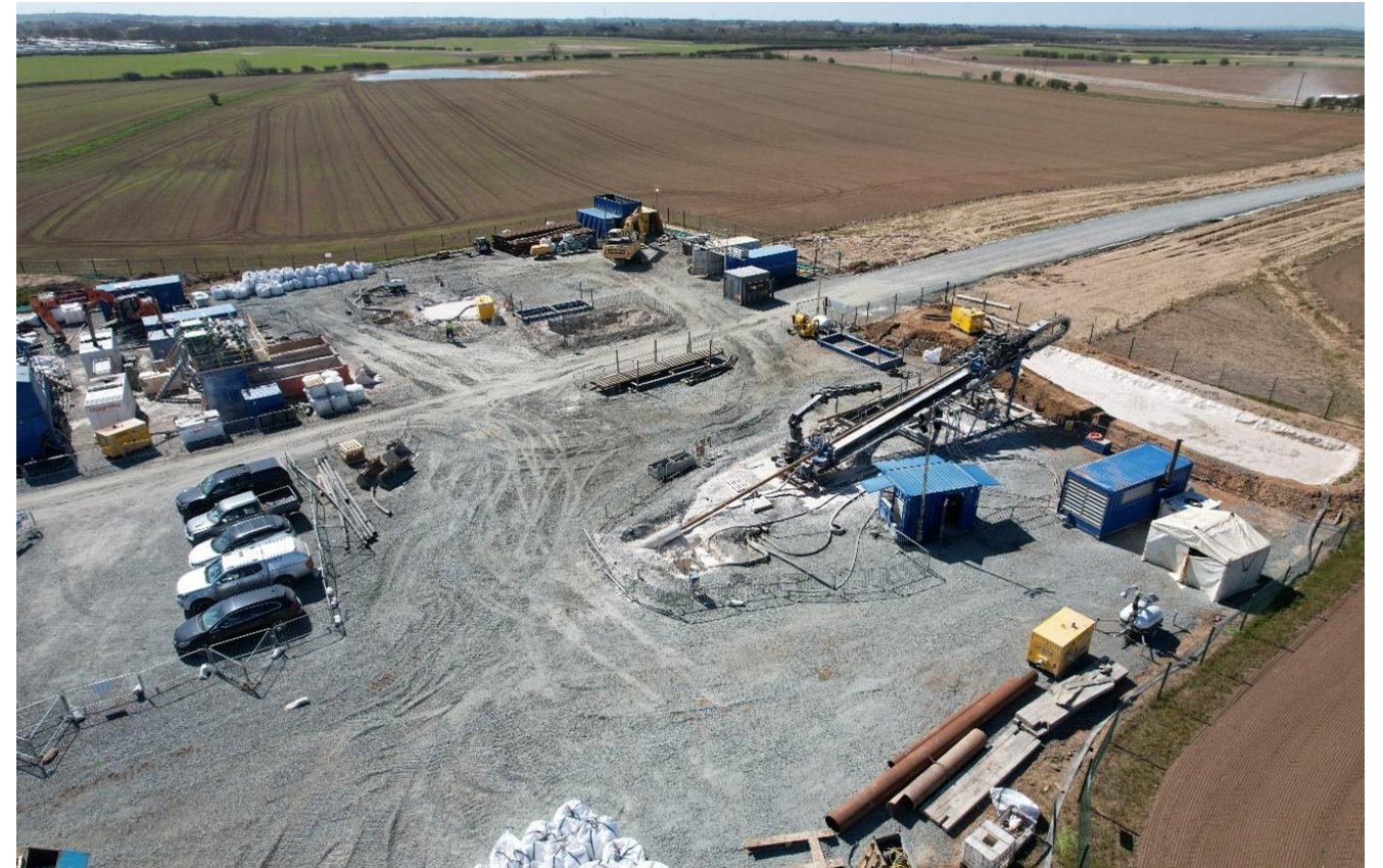
Plate 2-10 Example of a Landfall Construction Compound (Note: Compound will be dependent on the selected trenchless installation technique at landfall) (Source: Dogger Bank A & B)
