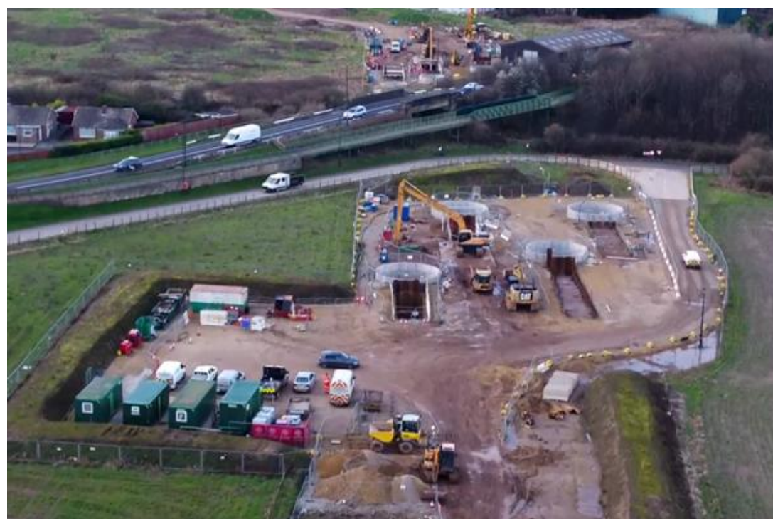
Plate 2-15 Example Trenchless Installation Compound for Onshore Export Cable Works (Note: Compound dependent on the selected trenchless installation technique at each crossing) (Source: Dogger Bank C)
